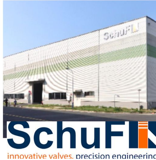
ASSEMBLY AND TESTING IN LEASED WORKSHOP 10.2023
